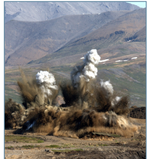
Aqqaluk first blast on June 8, 2010 at 12:14 p.m. Although small in size, the shot was huge in its representation that mining was underway.
